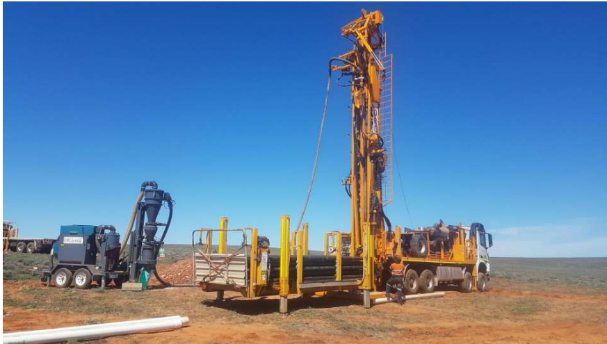
Figure 1: Drilling rig on site drilling the first hole on the Pernatty project area
