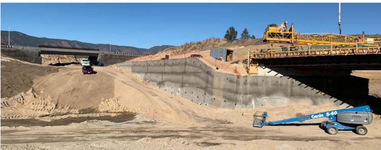
**Figure 4. Bridge embutment and retaining wall constructed with EdenCrete® enriched concrete**
