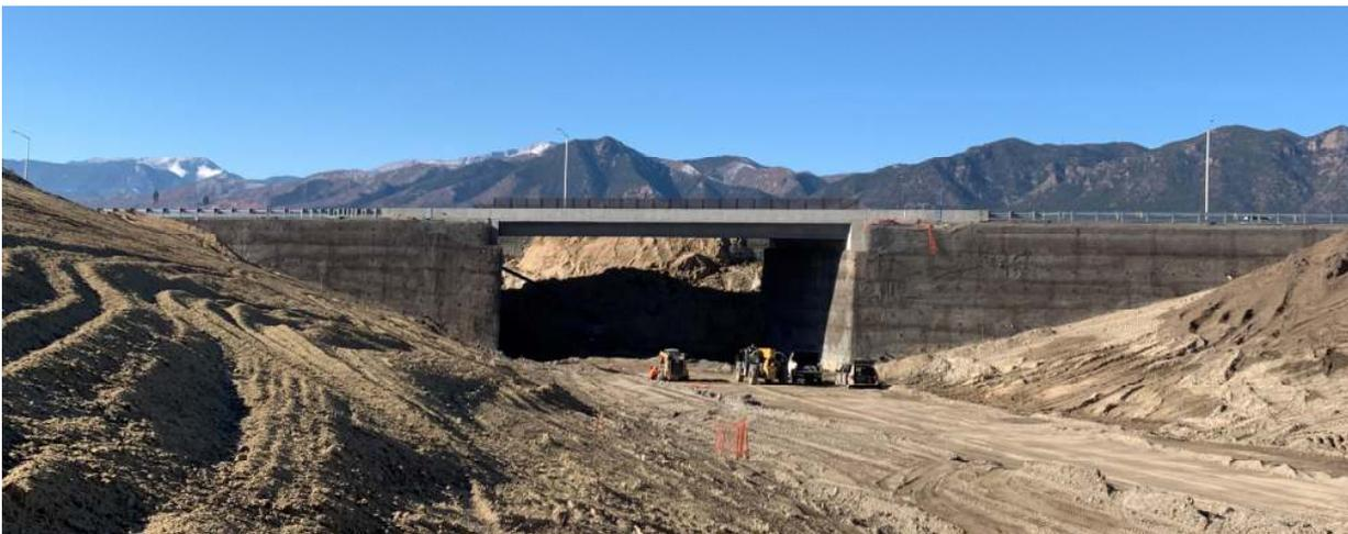
**Figure 3. Underpass, wing walls and embutment constructed with EdenCrete® enriched concrete**
