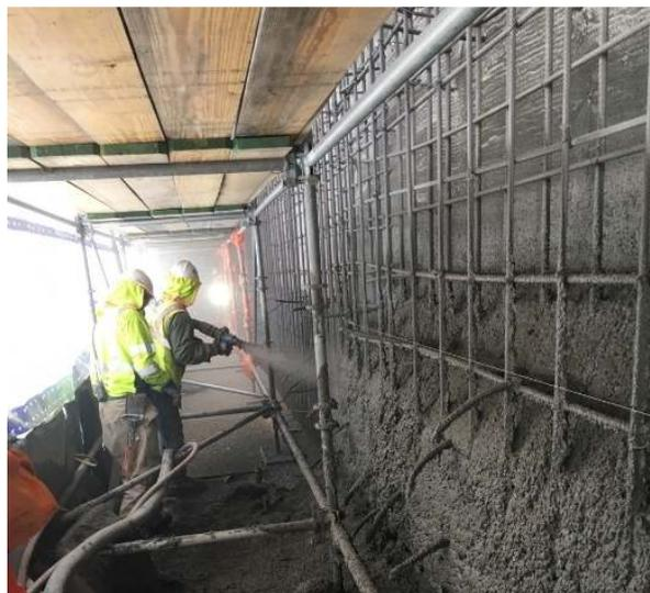
**Figure 4. The EdenCrete® enriched Shotcrete being applied**
