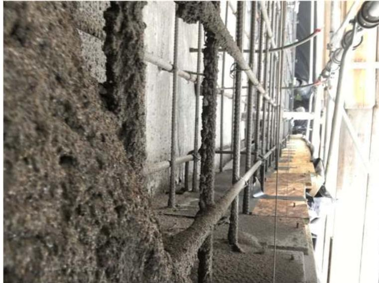
**Figure 5. Close - up photo of EdenCrete® Shotcrete**
