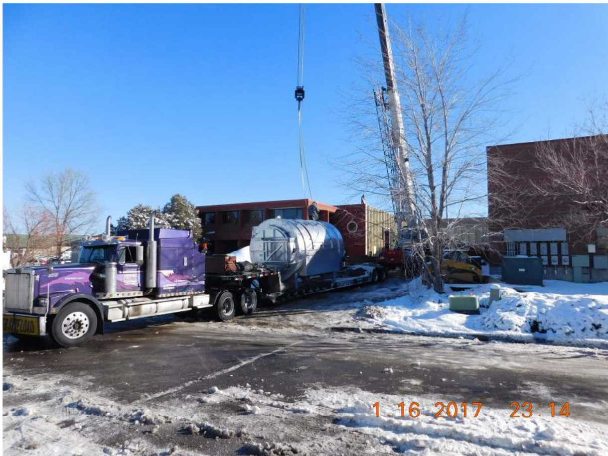
Figure 1. Reactor Being Lifted Off Low Loader.
