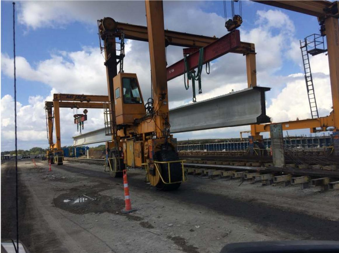
**Figure 1. Typical Precast / prestressed bridge beam being fabricated**
