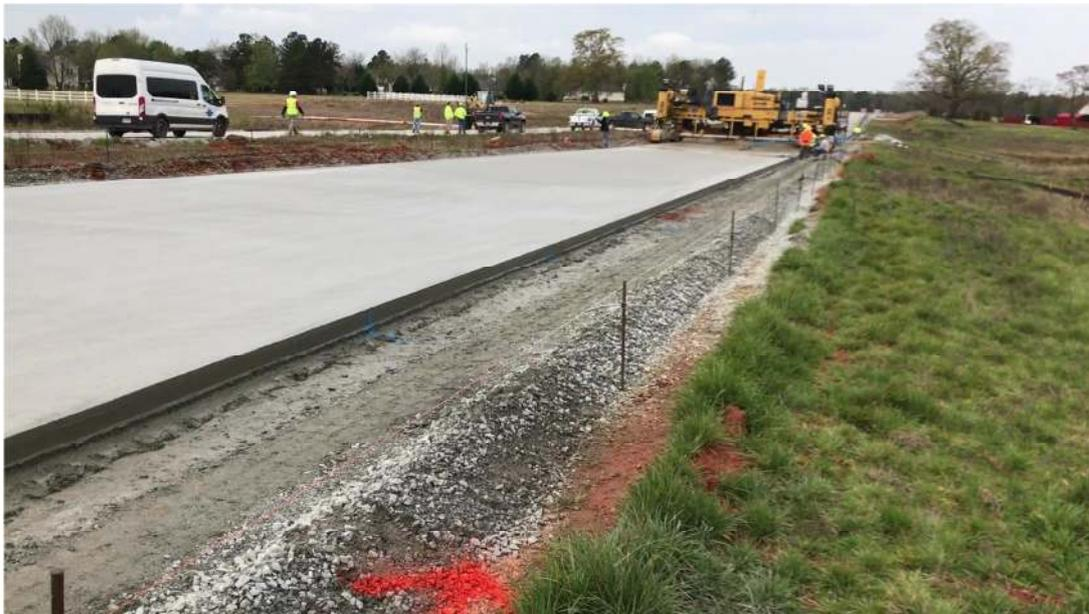
Figure 2. Completed section of highway with added EdenCrete<sup>®</sup>
