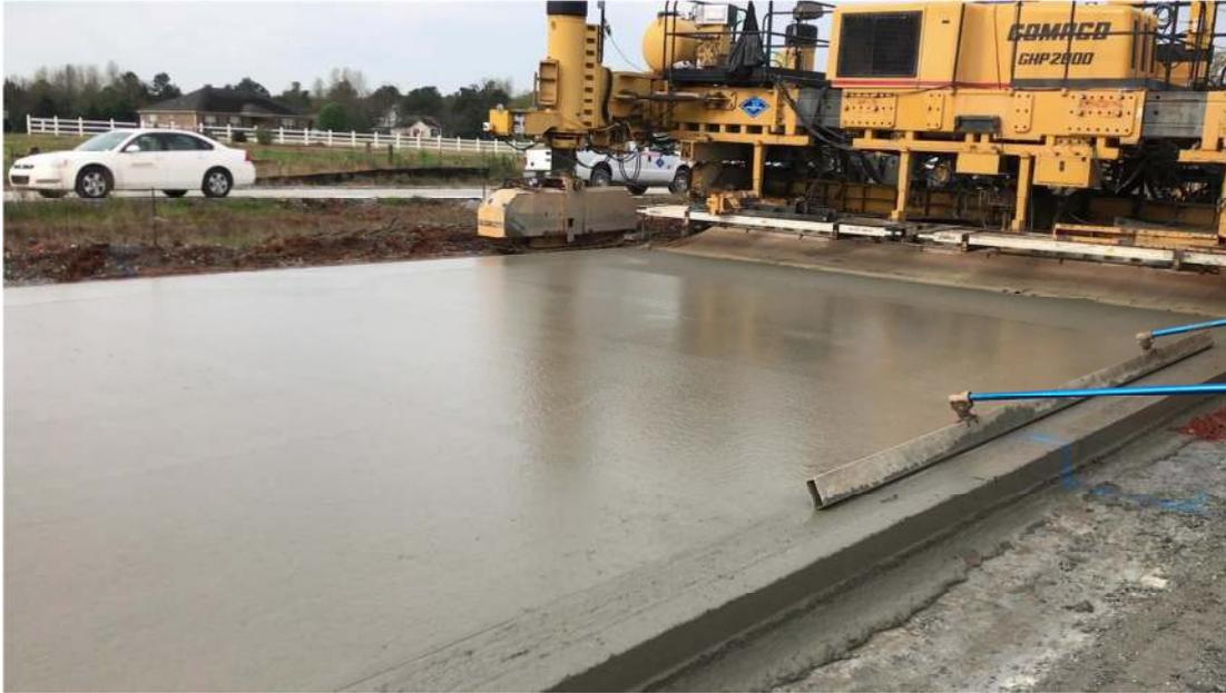
Figure 1. EdenCrete<sup>®</sup> - enriched concrete being laid in Field Trial
