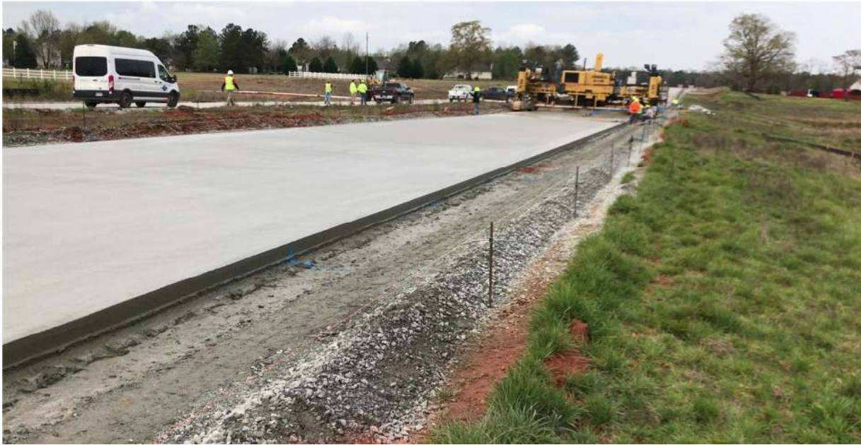
Figure 2. Completed section of new highway with added EdenCrete
