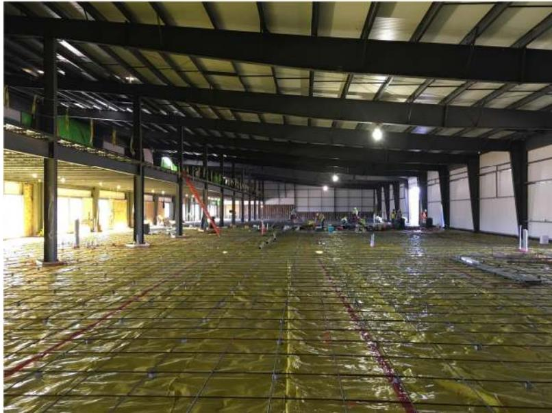
**Figure 1. New factory concrete floor being prepared**
