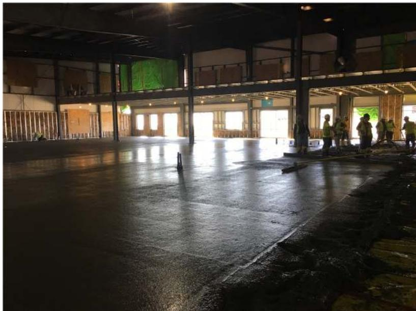
**Figure 2. New factory concrete floor being poured**
