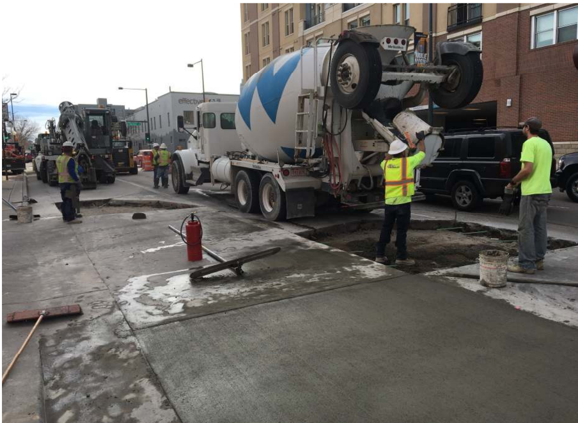
Figure 2. EdenCrete® Trial Slabs on 22 nd Street, Denver, Colorado.
