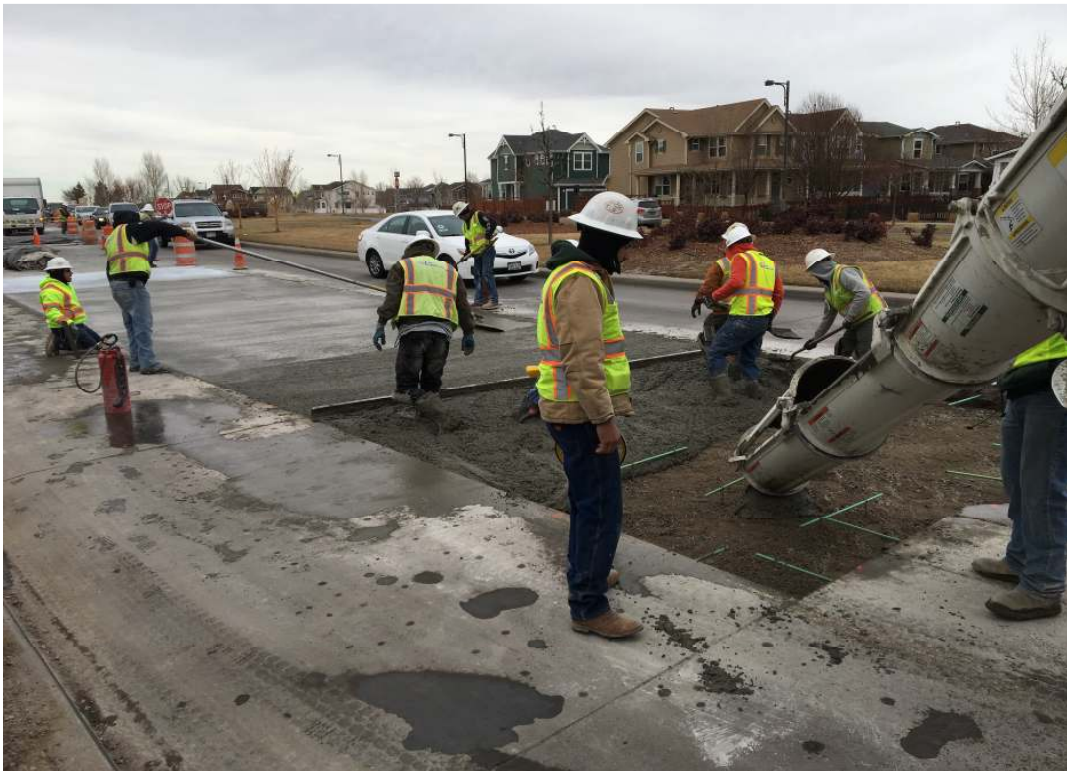
Figure 4. EdenCrete® Trial Slabs on Central Park Ave, Denver, Colorado.
