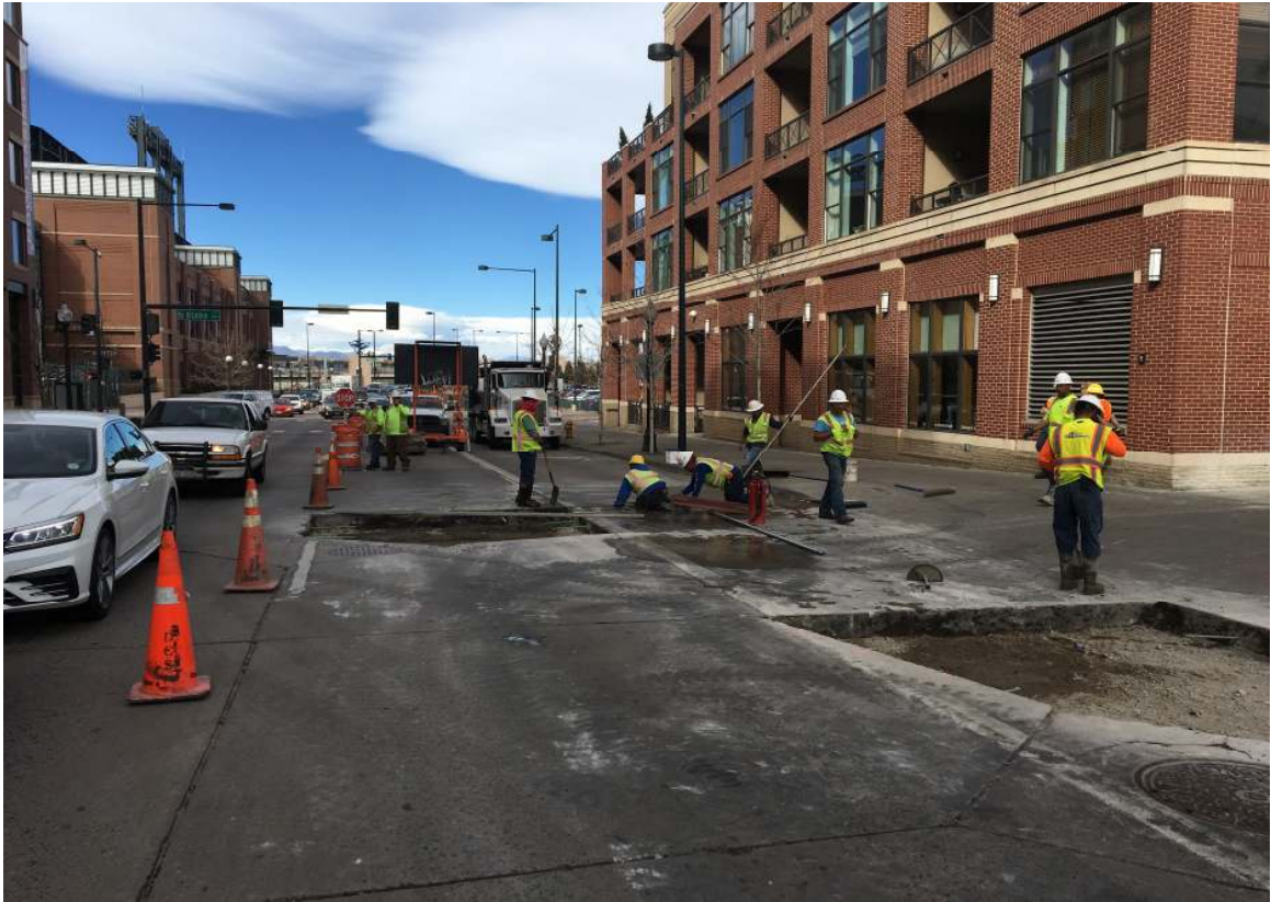
Figure 1. EdenCrete® Trial Slabs on 22 nd Street, Denver, Colorado.
